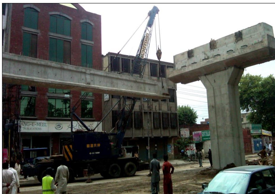
FIGURE 5.26: LAUNCHING OF I-GIRDER
