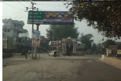
1. Absence of pedestrian facilities
