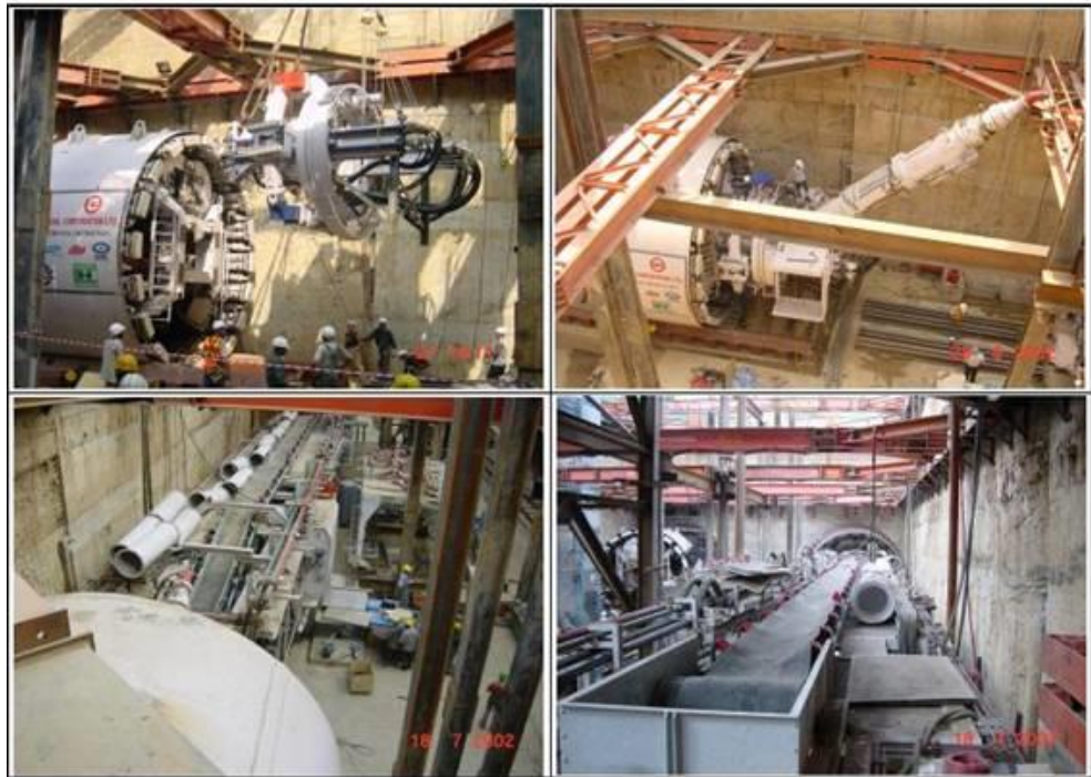
FIGURE 5.35: ERECTOR, SCREW CONVEYOR & BACKUP SYSTEM
