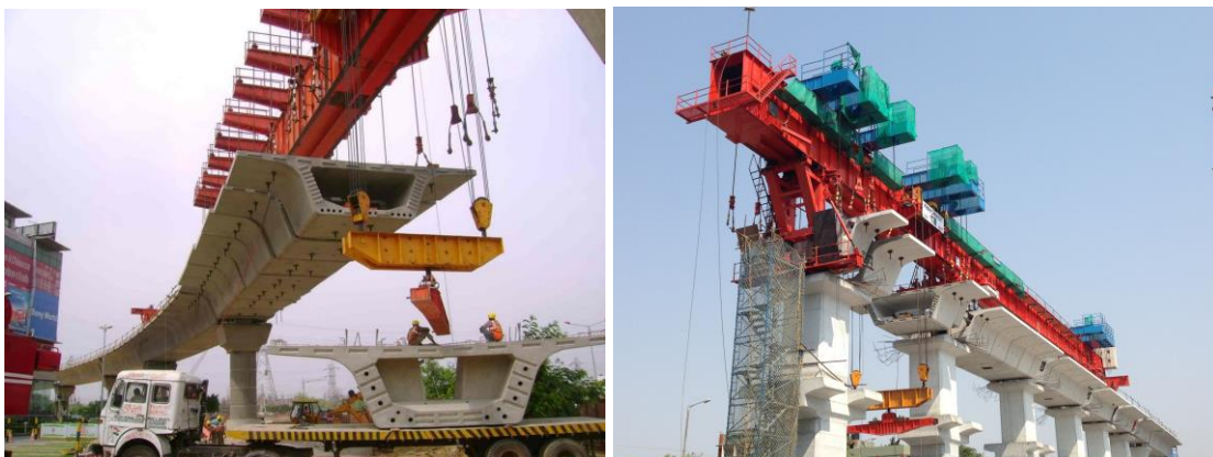
FIGURE 5.23: LAUNCHING OF BOX GIRDER SEGMENTS
