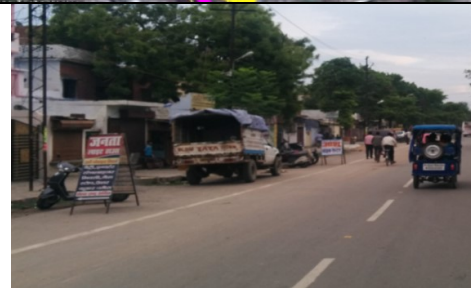
2. Encroachment of shoulder and footpath by vehicles
