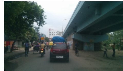
4. Ending of Flyover near Station Location
