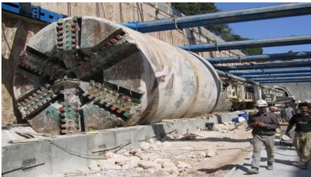
FIGURE 5.39: TBM PUSHED TO THE OTHER END OF THE STATION
