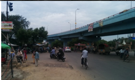
1. Absence of pedestrian facilities
