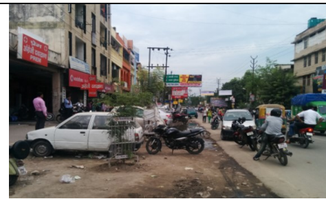
4. Encroachment of shoulder
