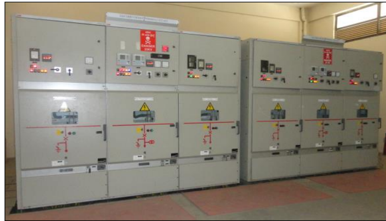
FIGURE 12.4: TYPICAL INDOOR AUXILIARY SUB-STATION (ASS)
