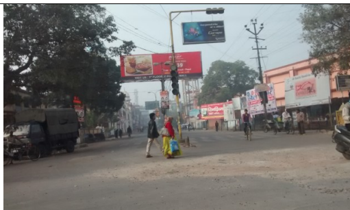
3. Road surface conditions are poor
