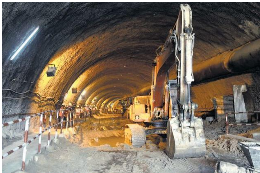
FIGURE 5.40: CONSTRUCTION OF TUNNEL BY NATM
