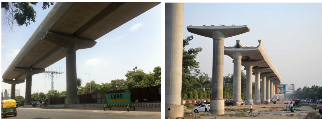
FIGURE 5.24: PRECAST U-CHANNEL SUPERSTRUCTURE
