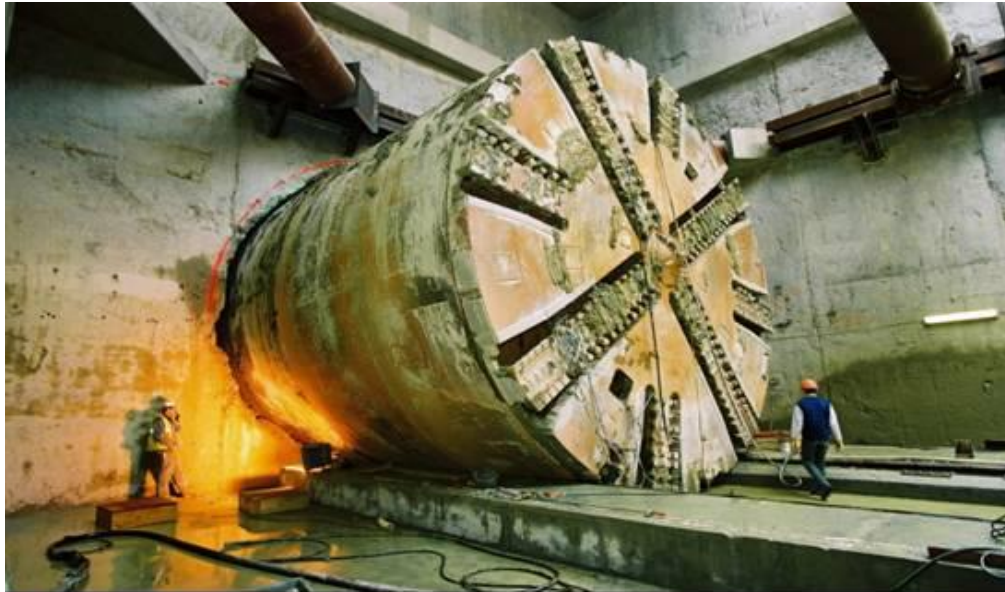
FIGURE 5.39: TBM PUSHED TO THE OTHER END OF THE STATION
