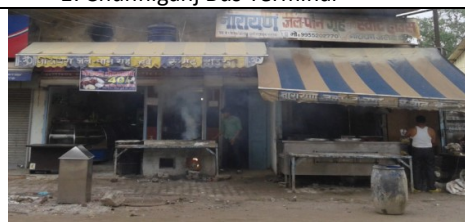
3. Absence /discontinuous/ encroached footpath
