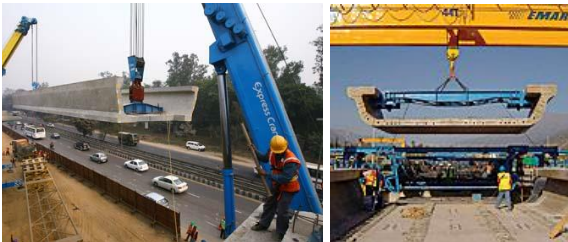
FIGURE 5.25: LAUNCHING OF U-CHANNEL GIRDER
