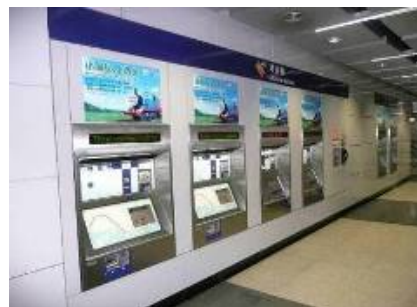
MTR Wall mounted TVM with maintenance corridor in the back – Paris
