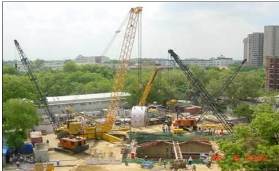
FIGURE 5.34: MAIN SHIELD ERECTION
