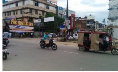
2. Absence of pedestrian facilities on cross roads
