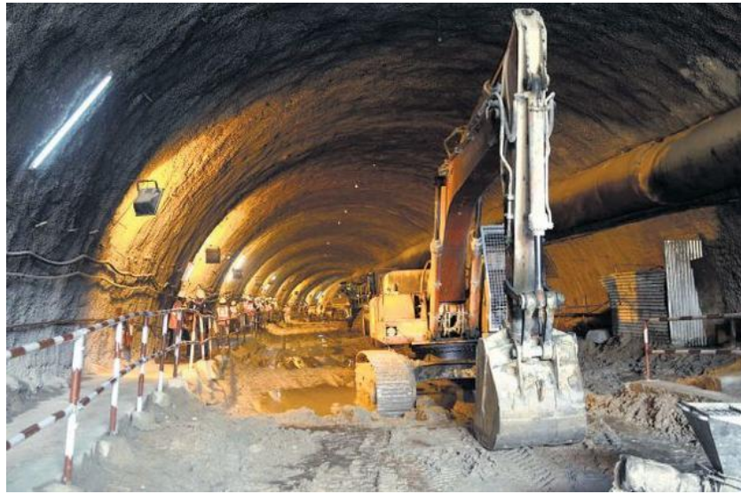
FIGURE 5.37: CONSTRUCTION OF TUNNEL BY NATM
