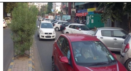
3. On-Street parking & Encroachment causes loss of efficient carriageway.
