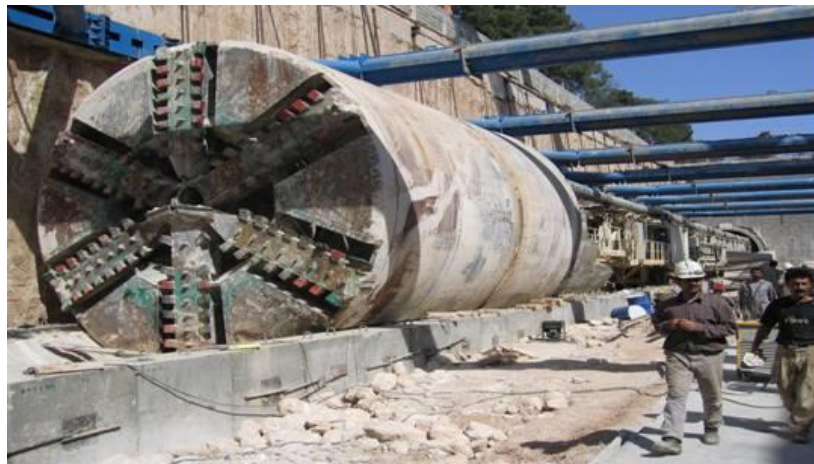
FIGURE 5.36: TBM PUSHED TO THE OTHER END OF THE STATION
