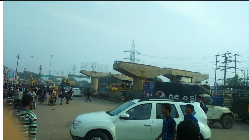
Under construction flyover at Water Works Chauraha near Lal Masjid
