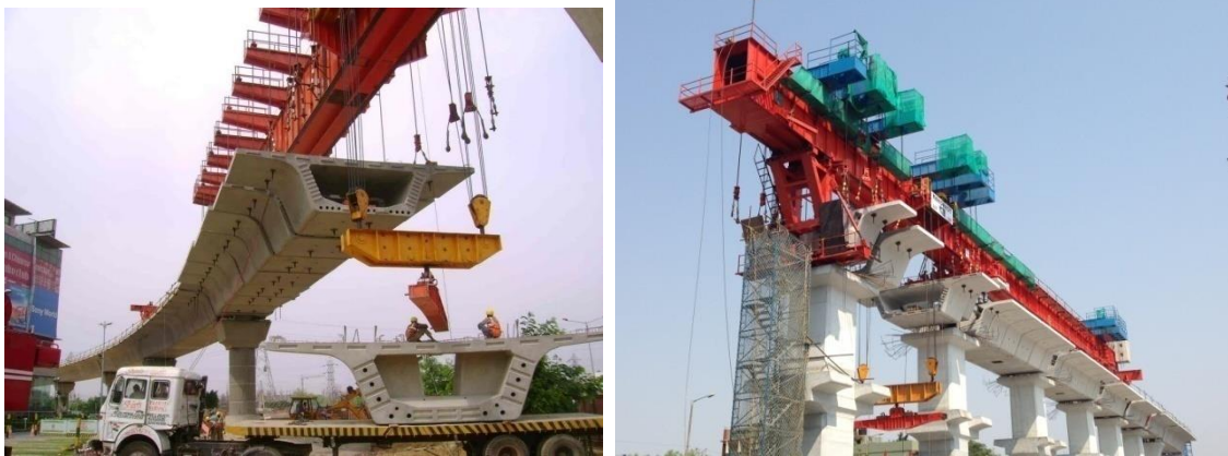
FIGURE 5.20: LAUNCHING OF BOX GIRDER SEGMENTS
