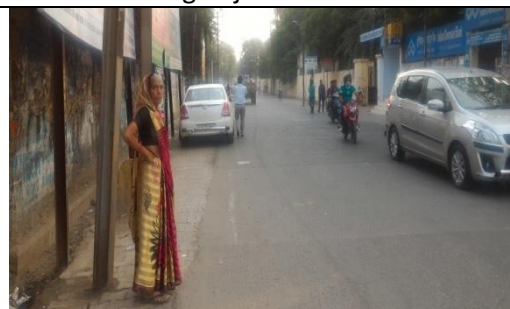
4. Narrow road width and absence of footpath.
