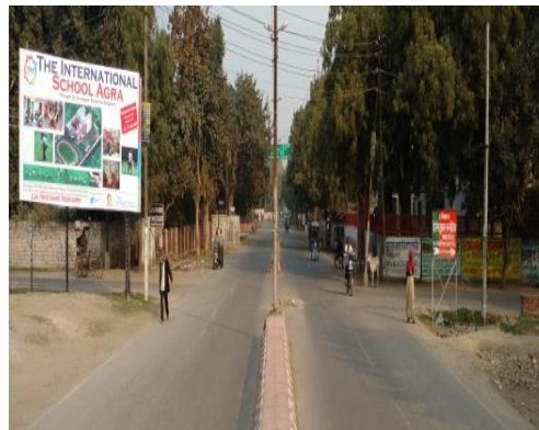
2. Absence of footpath, lack of pedestrian facilities.
