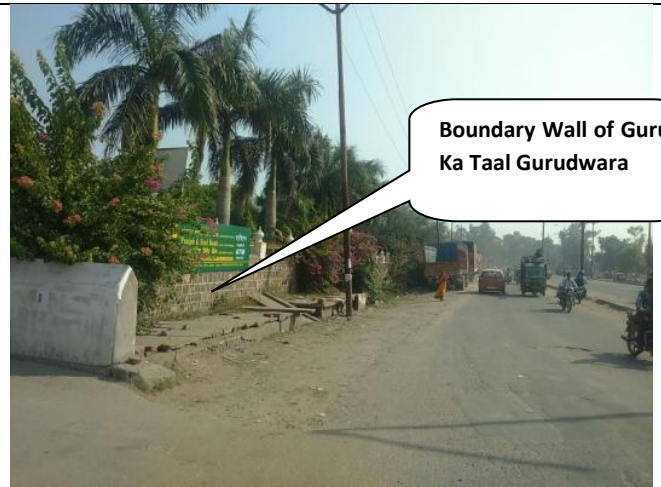
Boundary Wall Of Guru Ka Taal Gurudwara
