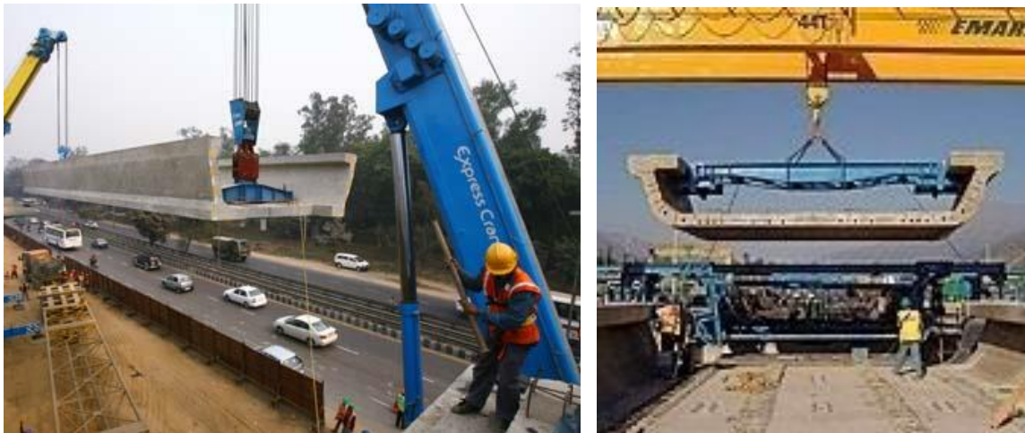
FIGURE 5.22: LAUNCHING OF U-CHANNEL GIRDER
