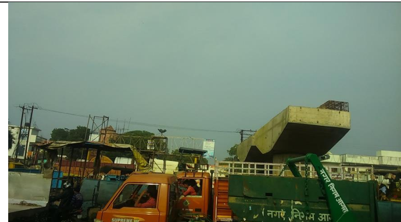
Under construction flyover at Water Works Chauraha near Lal Masjid
