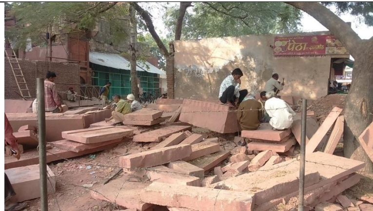
Maintenance work of Lal Masjid is in progress
