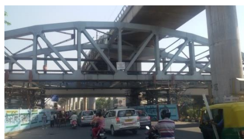
FIGURE 5.24: CLC SPAN 75M + 105M + 75M AND STEEL SPAN 60M
