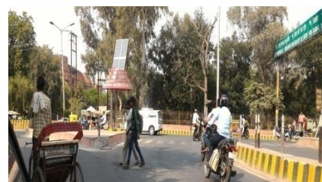
4. Lack of Pedestrian facilities.
