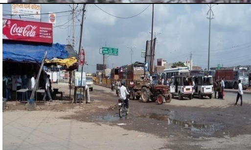
1. Poor conditions of road surface.
