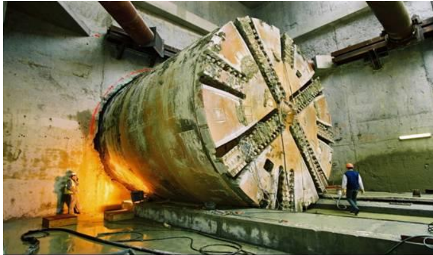
FIGURE 5.36: TBM PUSHED TO THE OTHER END OF THE STATION
