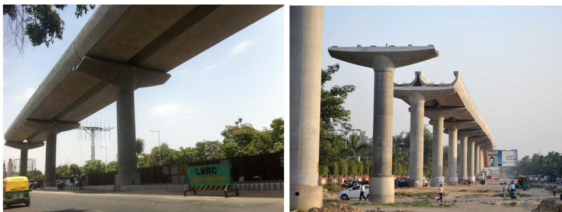
FIGURE 5.21: PRECAST U-CHANNEL SUPERSTRUCTURE
