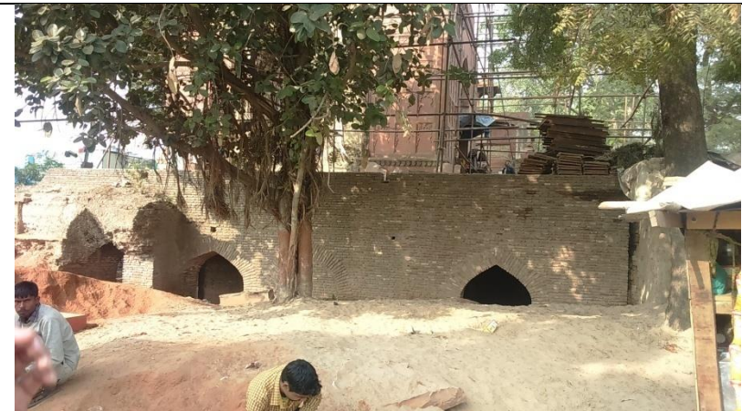
Maintenance work of Lal Masjid is in progress
