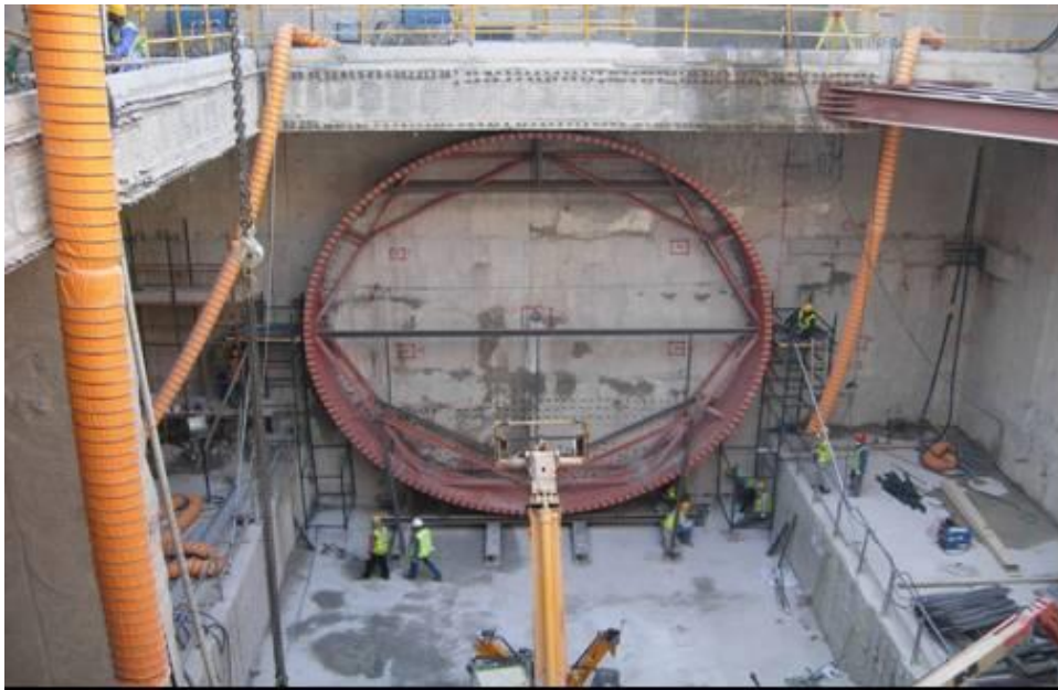
FIGURE 5.30: TYPICAL ASSEMBLY OF TUNNEL BORING MACHINE
