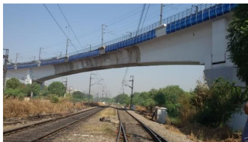
FIGURE 5.24: CLC SPAN 75M + 105M + 75M AND STEEL SPAN 60M
