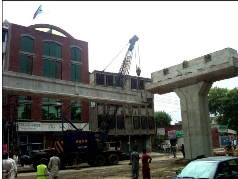
FIGURE 5.23: LAUNCHING OF I-GIRDER
