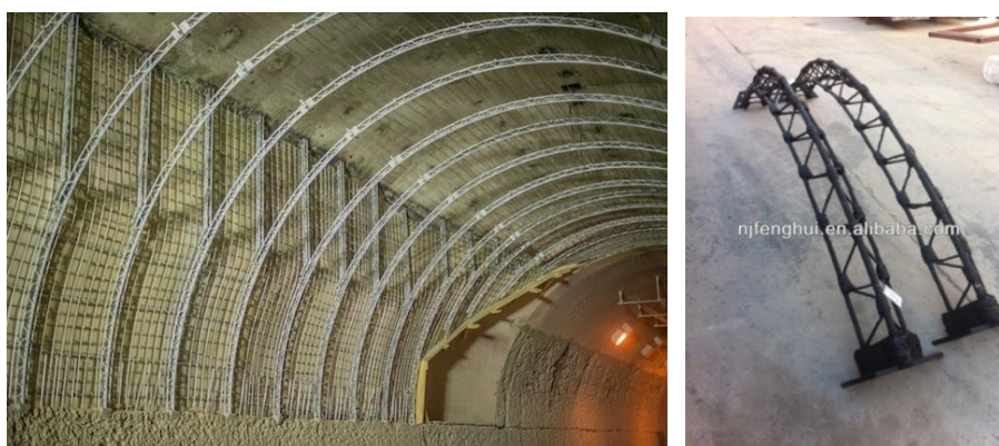
FIGURE 5.39: LATTICE GIRDER
