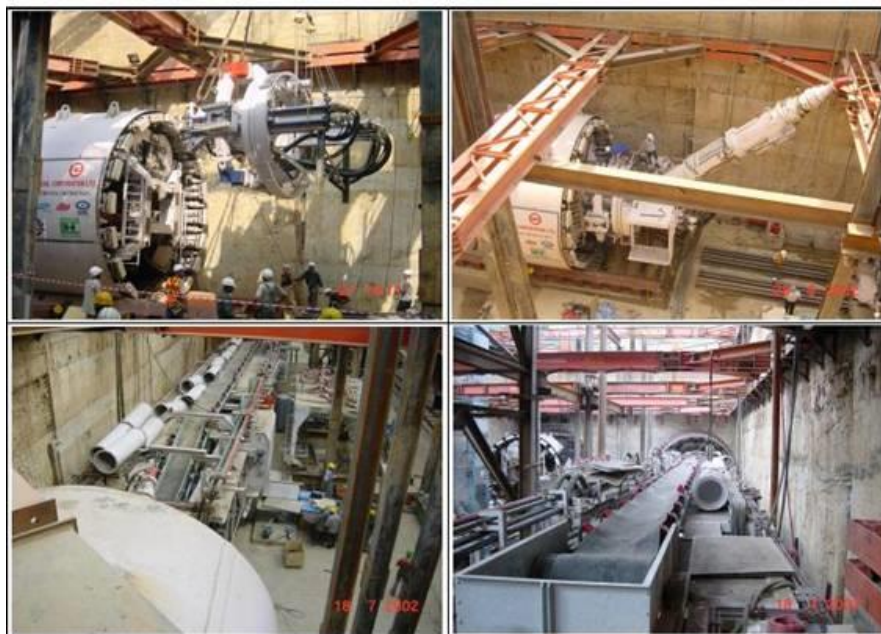
FIGURE 5.32: ERECTOR, SCREW CONVEYOR & BACKUP SYSTEM
