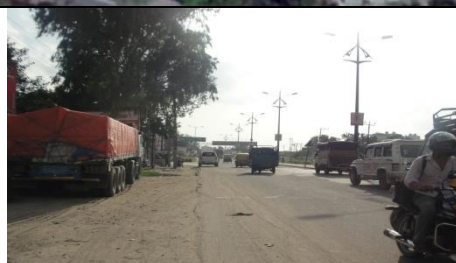
2. On-street parking of heavy vehicles reduces road width.
