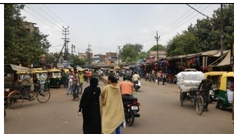
4. Absence/discontinuity of footpath, lack of pedestrian facilities.
