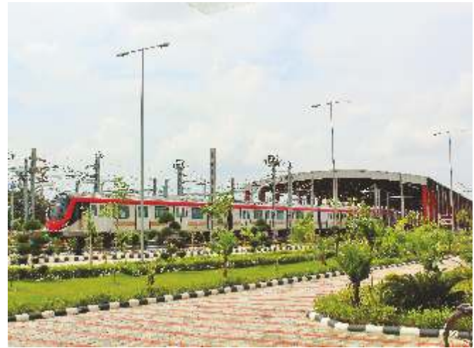
Metro Train at the Stabling Yard Inside Green Depot
